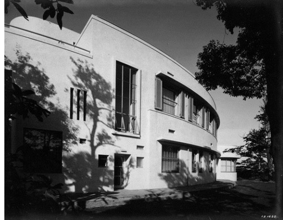
Exterior view of the south facade
