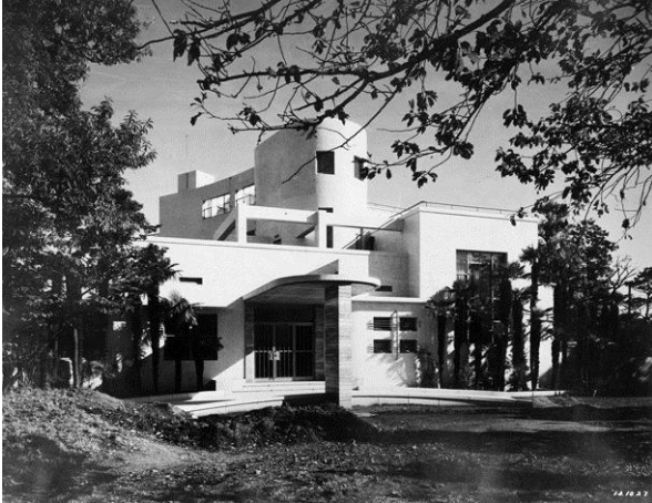
Exterior view of the entrance
